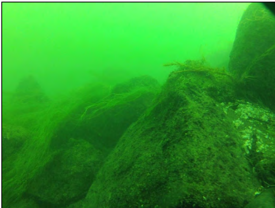
FIGURE 3. ROCK WING STRUCTURE UPSTREAM OF THE SOUTH GRAND ISLAND BRIDGE
